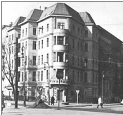
War damages: turret and stucco are gone
